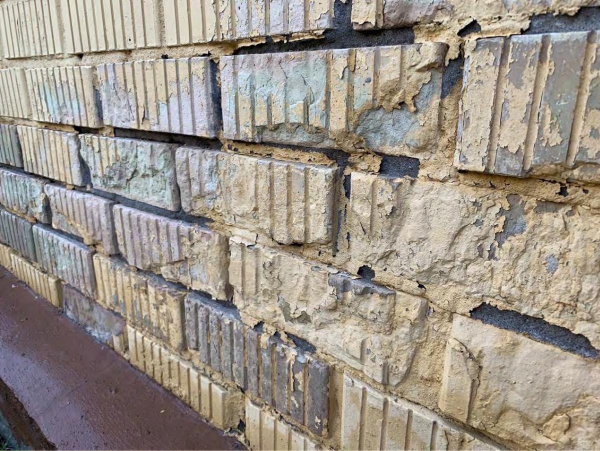
Due to significant power surges, the electrical system has experienced a failure. Unfortunately, this has led to power outages, preventing us from properly heating the house. Consequently, the walls have become frozen and damp, resulting in the development of cracks throughout the façade. Additionally, the old roof and fence are also in need of repair.
