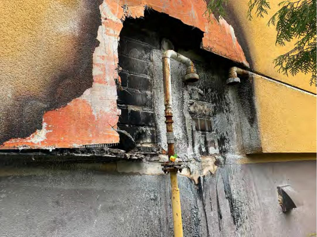
With the start of severe power outages in the winter of 2022-2023, the wiring, which has been over 20 years old, could not withstand the voltage. A fire broke out at the intersection of the gas and electrical wiring which led to the fire of the gas pipe and part of the house facade.
