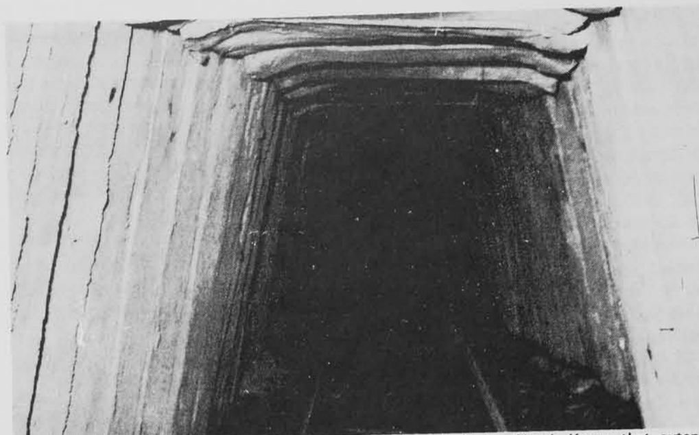
This photo shows part of a concrete-reinforced tunnel built by North Korea that extends two-thirds of a mile into South Korean territory. It is large enough to send through an entire regiment in an hour to stage a big-scale surprise attack.
