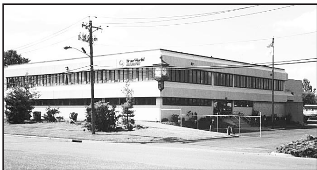
True World Marine boat building factory in Little Ferry
