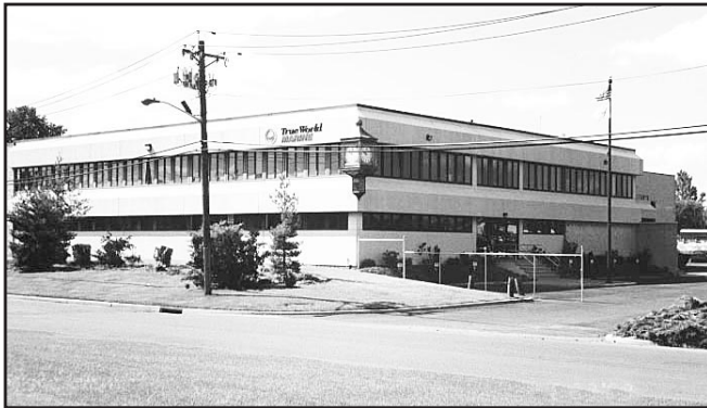
True World Marine boat building factory in Little Ferry
