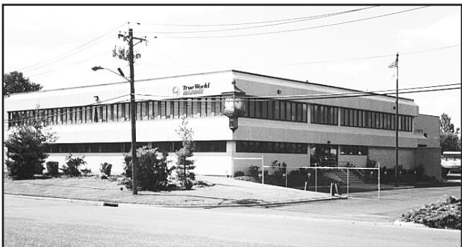
True World Marine boat building factory in Little Ferry
