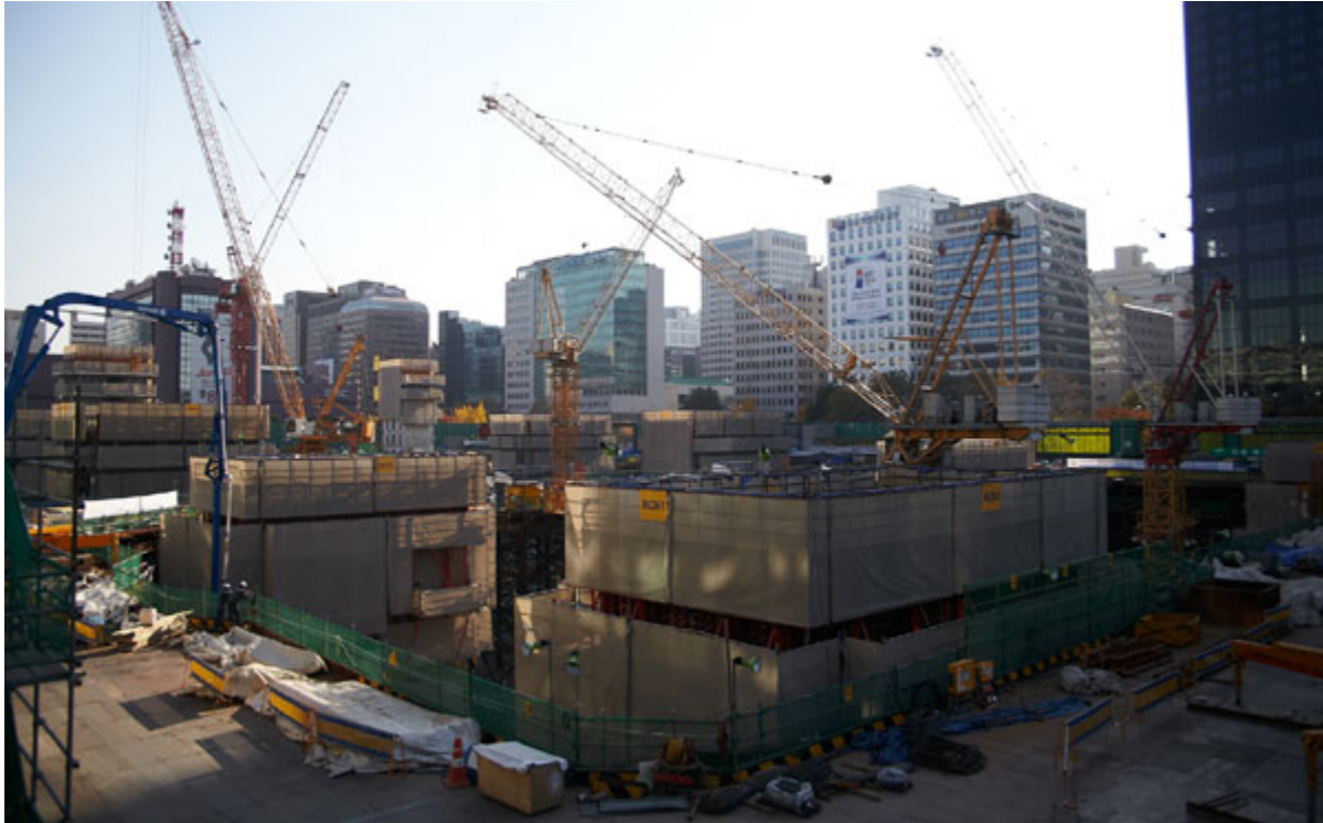
(Photo: The Parc 1 construction site at 22 Yeouido-dong Youngdungpo-ku, Seoul. The construction came to a halt in the beginning of November.)
