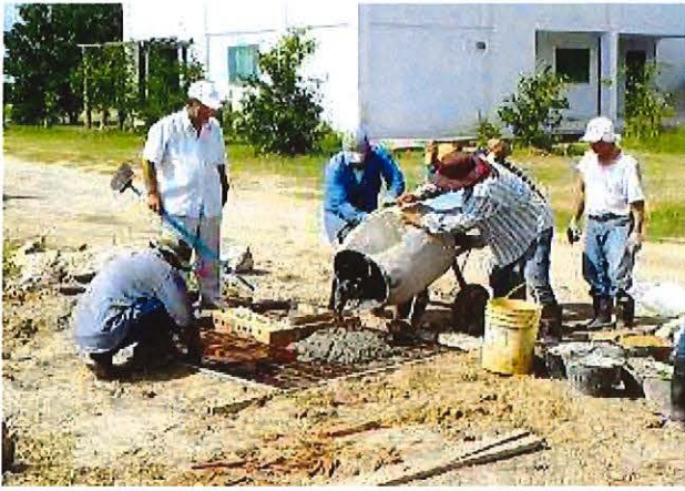
Construction of drainage for Capybara Land. Mr. Nakata (standing left) and Mr. Oyama (right)
