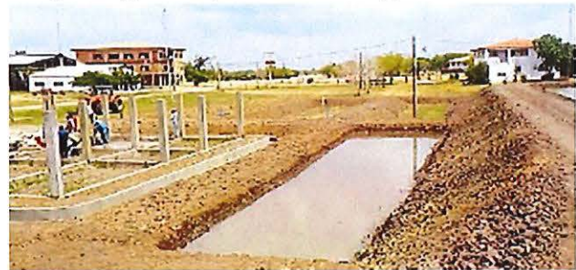
Preparing for 3 ponds in the ground.
