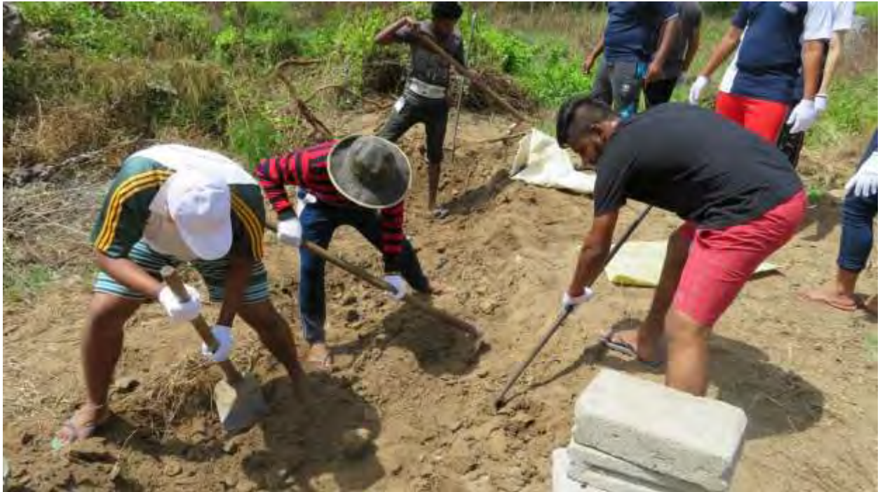
The hardworking RYS participants leveling the ground and securing the perimeter of the community center
