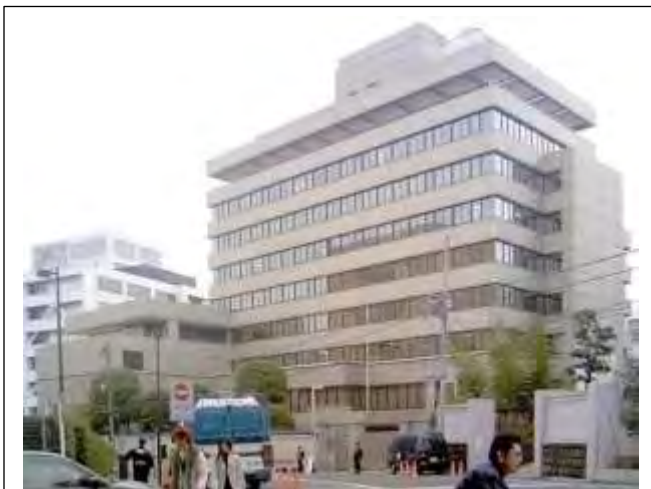
The Japanese headquarters of Chosen Souren (General Association of North Korean Residents in Japan) in Chiyoda, Tokyo, Japan. Photo: GcG / Wikimedia Commons
