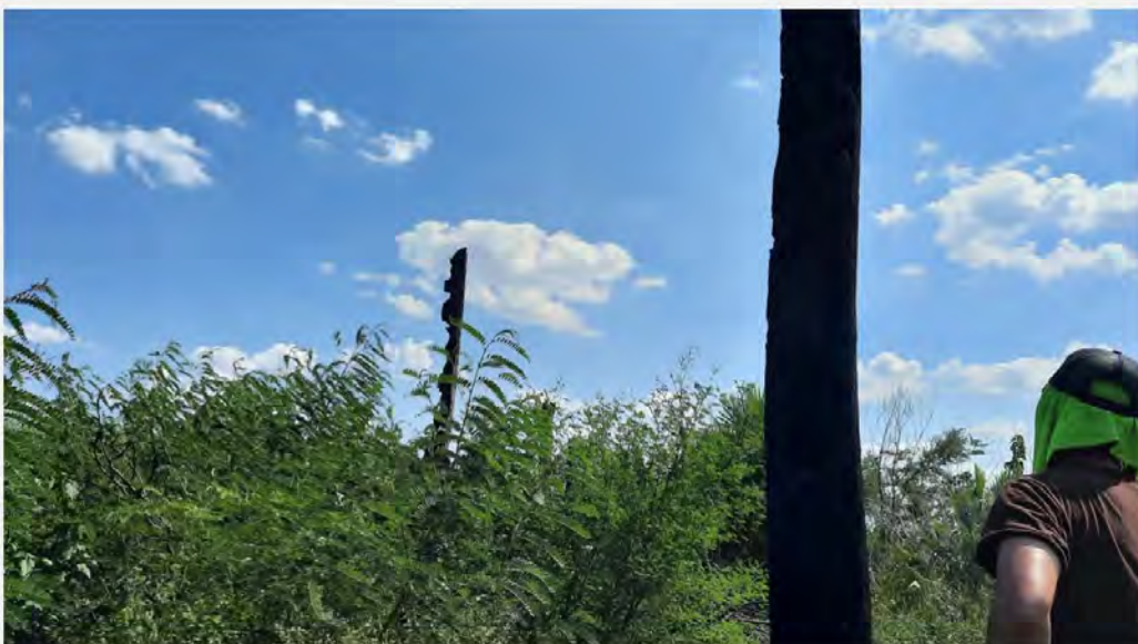
Looking at one still-standing pillar of what used to be room 14
