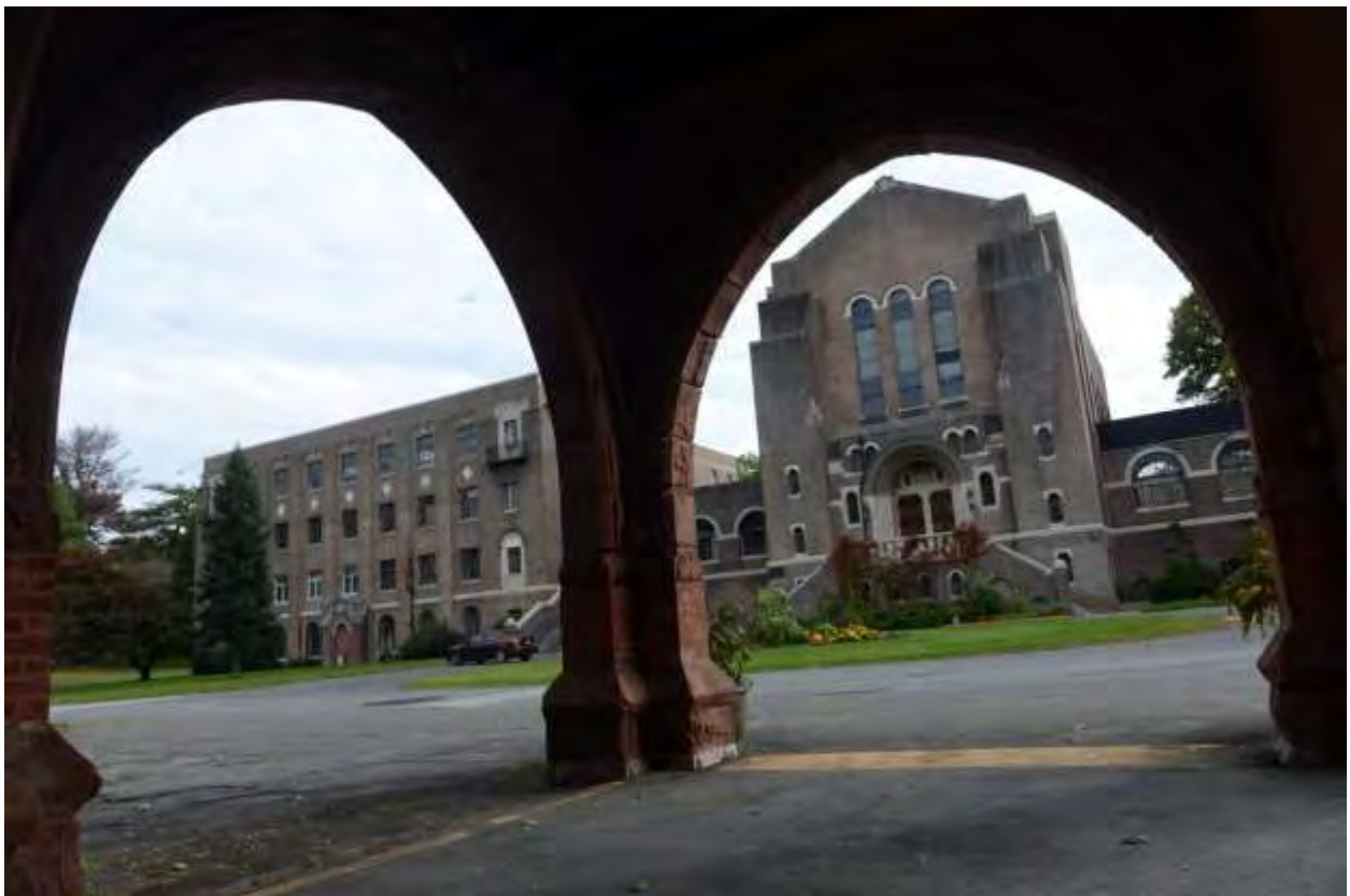
One of the buildings that was once home to the Unification Theological Seminary in Barrytown, N.Y.
