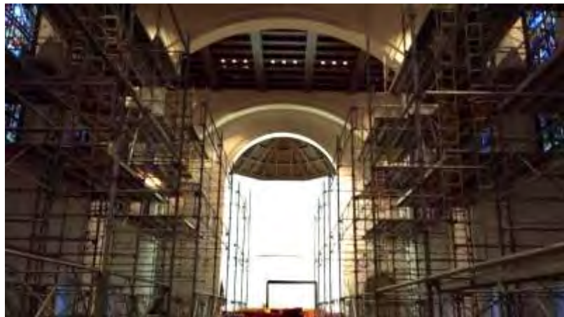
Scaffolding in UTS Chapel for Window Replacement
