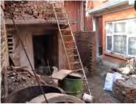
Rear of our apartment. (Owner is building a room for a security person to protect us against thieves).
