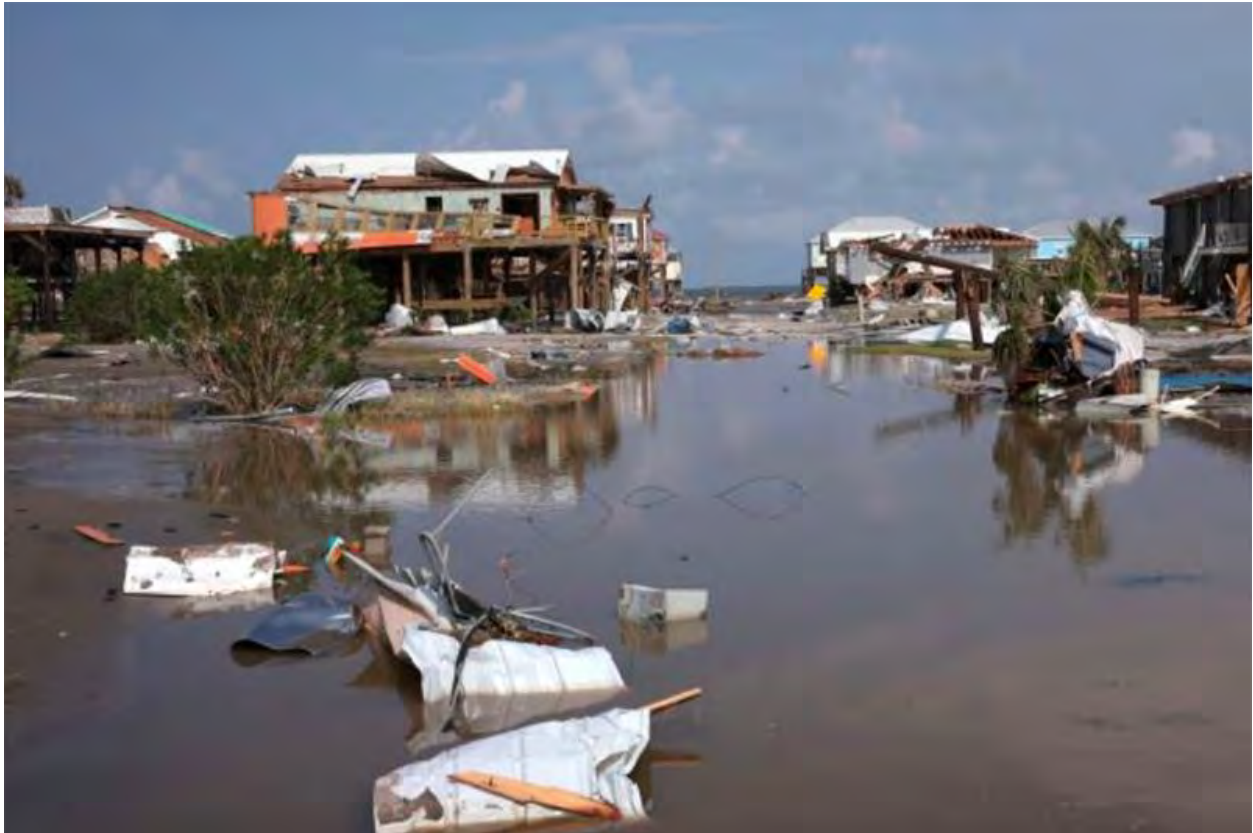
Flooding from Hurricane Ida in coastal Louisiana
