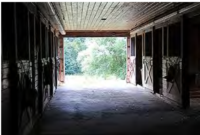
View from inside the stable
