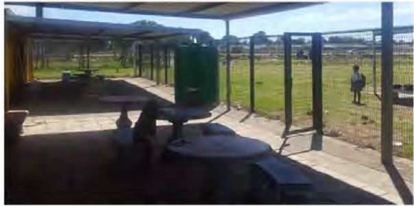
The finished fence
