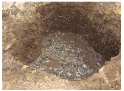
Not to be deterred, several volunteers jumped back into the holes and filled buckets with water and wet soil. Water seepage was not going to stop them! Yet, despite their best efforts, it did not take long for the volume of muddy soil removed to be replaced by an equal volume of water. Frustration was growing because we needed to dig wide holes to the depth of eight feet as a foundation to install a hand drill.
