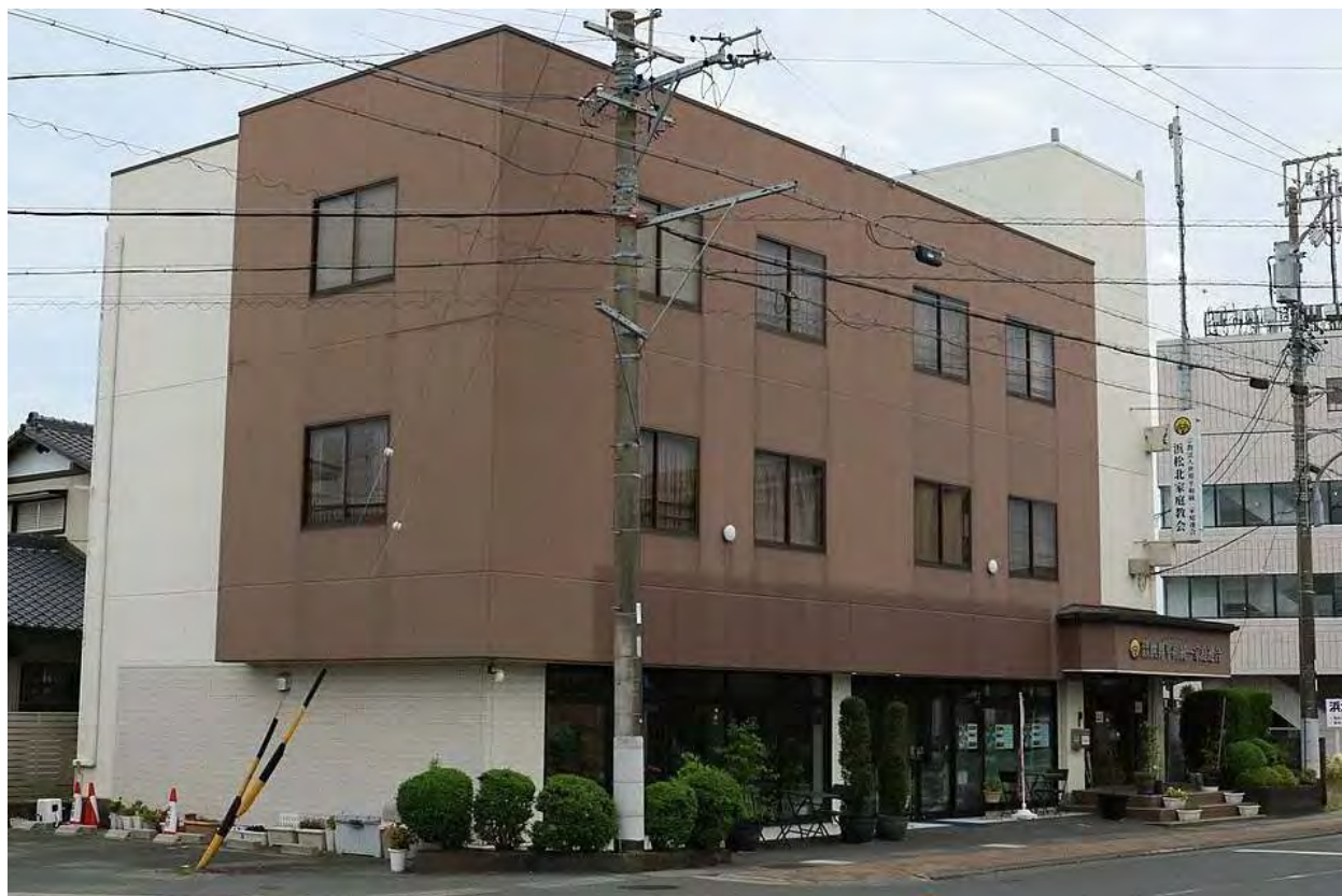
No more access to hundreds of its own buildings: Here, the property housing the Family Federation in North Hamamatsu, a city on the South coast on the main island of Honshu, Japan
