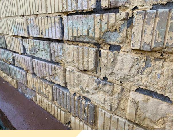
Due to significant power surges, the electrical system has experienced a failure. Unfortunately, this has led to power outages, preventing us from properly heating the house. Consequently, the walls have become frozen and damp, resulting in the development of cracks throughout the façade. Additionally, the old roof and fence are also in need of repair.
