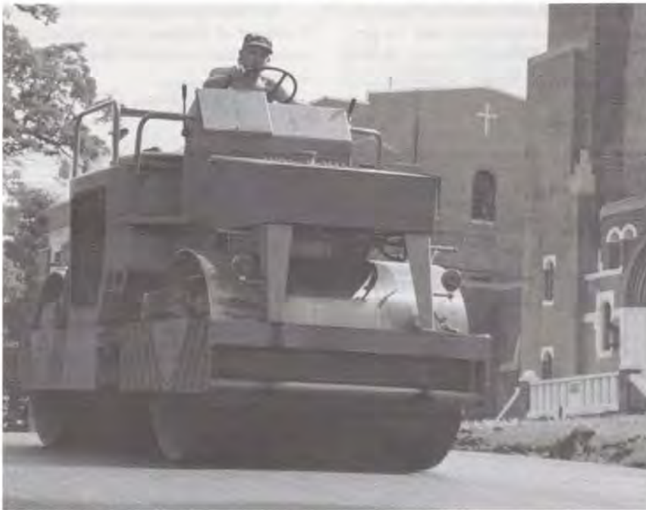
Rhinebeck Escavating's heavy roller puts the finishing touches on UTS' new driveway.
