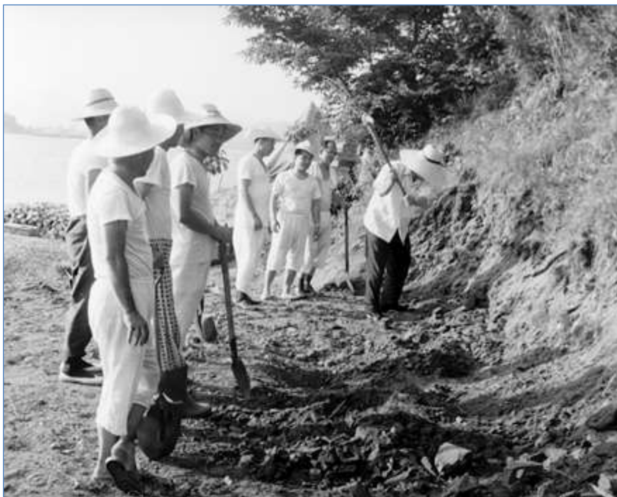
1971. 6. 17. True Parents pickaxing the ground as they work on the foundation of the Original Sanctuary
