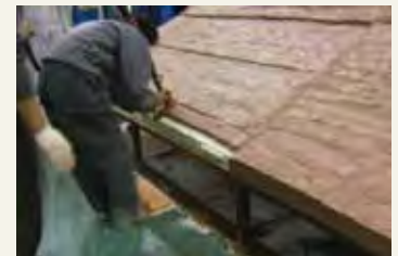
Automatic application of resin plaster
