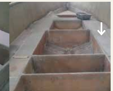
Sealing up the bulkheads
