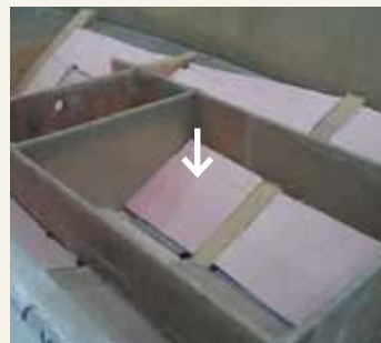
Laminate using two layers of urethane foam for reinforcement
