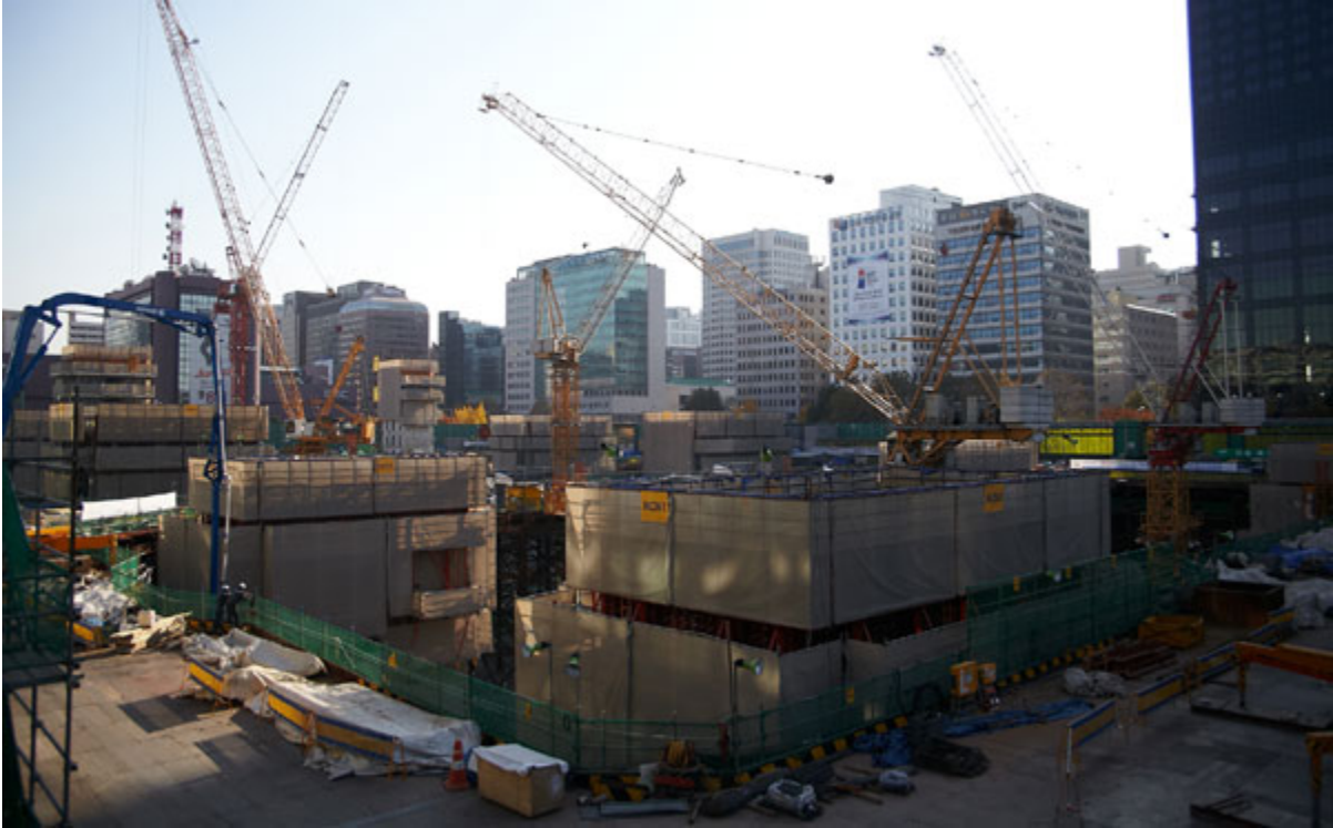
(Photo: The Parc 1 construction site at 22 Yeouido-dong Youngdungpo-ku, Seoul. The construction came to a halt in the beginning of November.)
