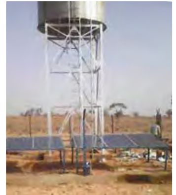
Water Tower with Solar Panels
