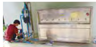
Installed Water Purifier and Water Fetching Place
