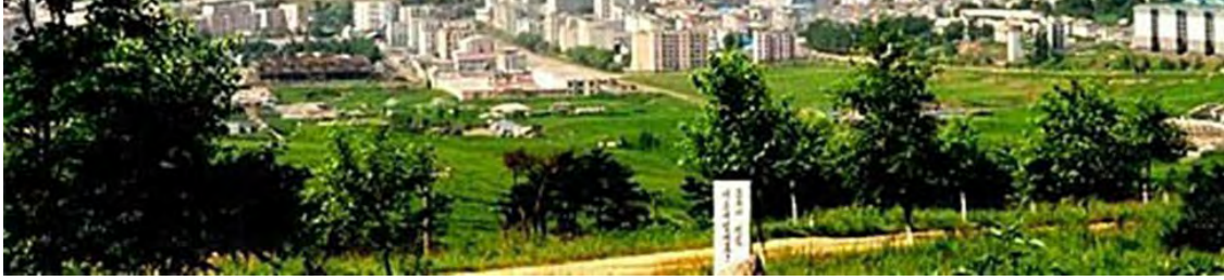
Factories and other buildings in Rason Special Economic Zone. [Source: reddit.com ]
