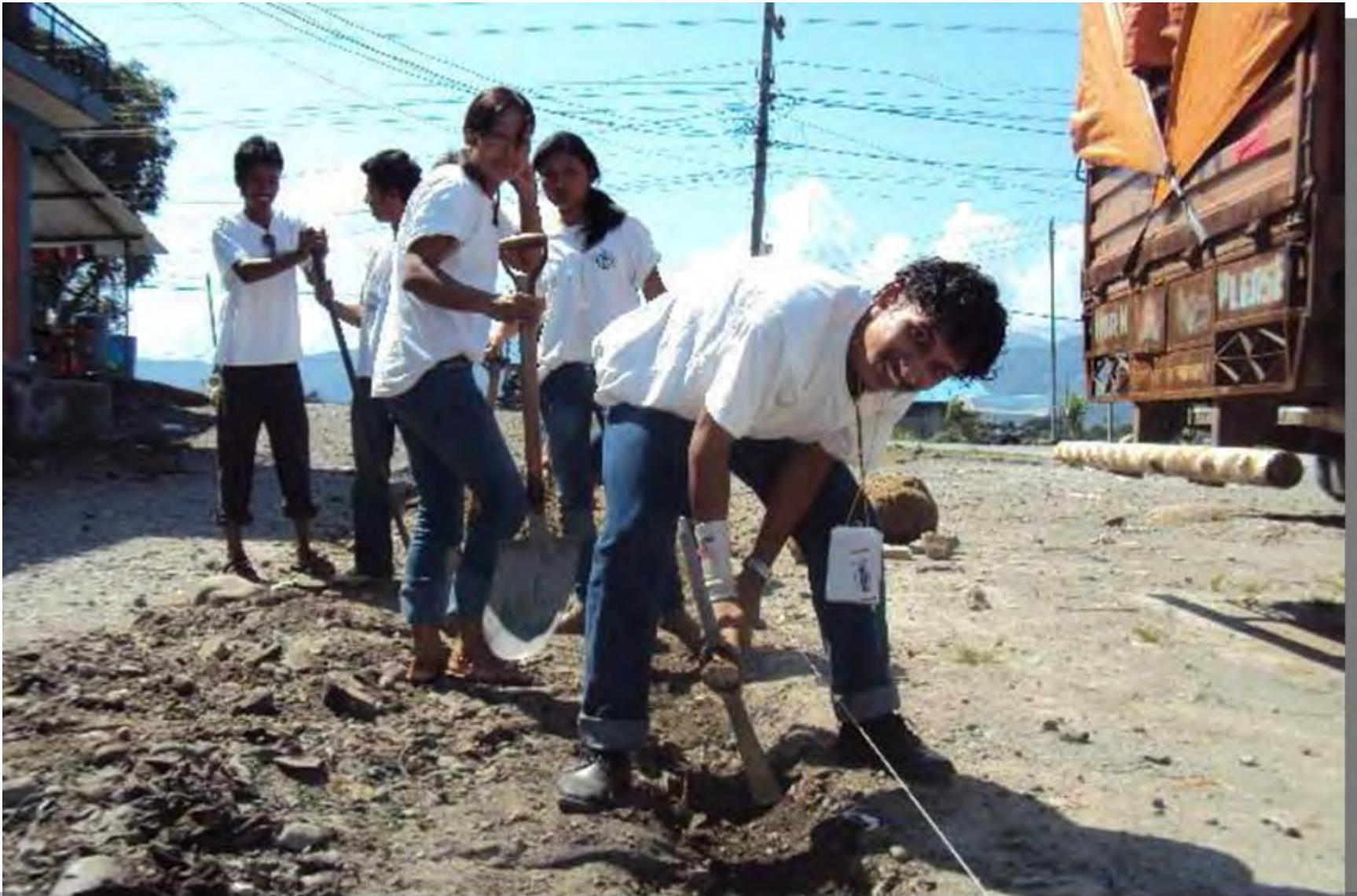
Pokhara, Nepal: Volunteers upgrade the landscaping at a local school.
