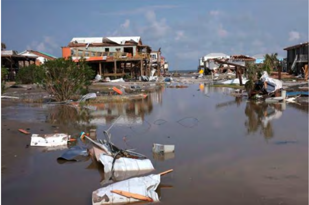
Flooding from Hurricane Ida in coastal Louisiana
