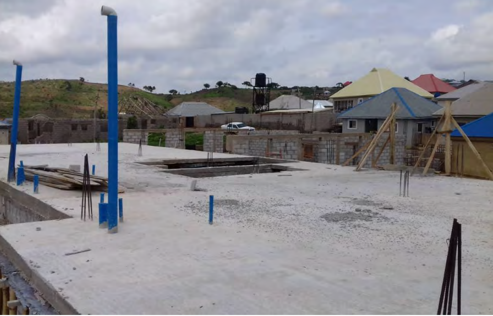
Finished decking for the office and Sunday School halls
