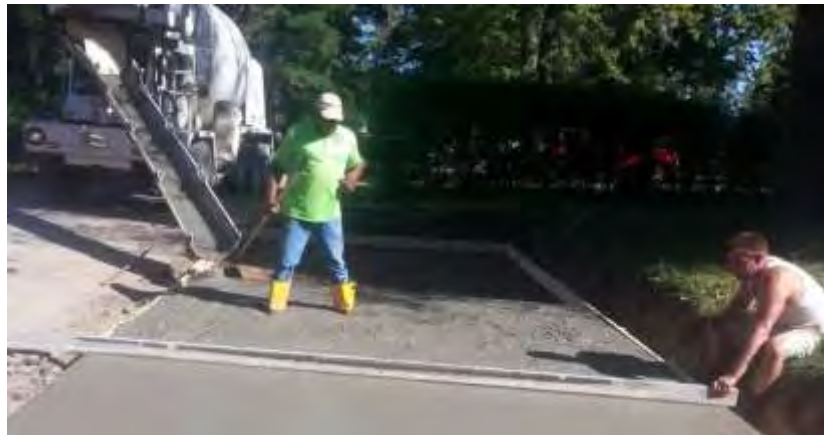
Paving in Barrytown this week
