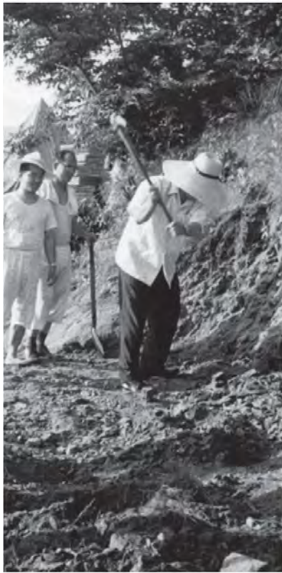
Construction of the Cheongpyeong Training Center began on June 17, 1971.
