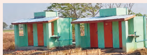
Completed school toilets
