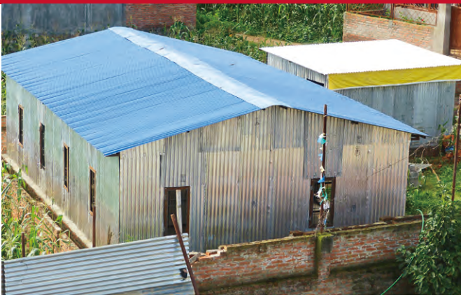
Newly built shelter with donation from WFPW Japan
