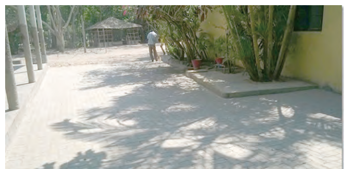
Block paved passage
