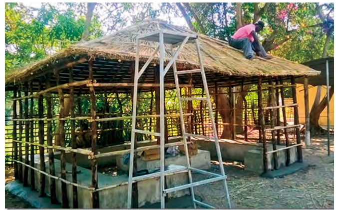
Renovation of arbor
