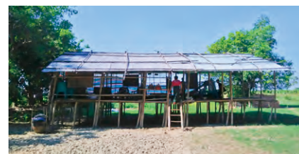
Temporary school building villagers built
