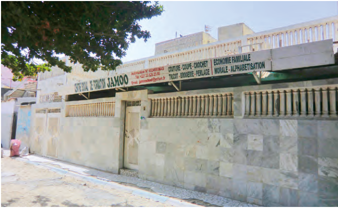
Current school building
