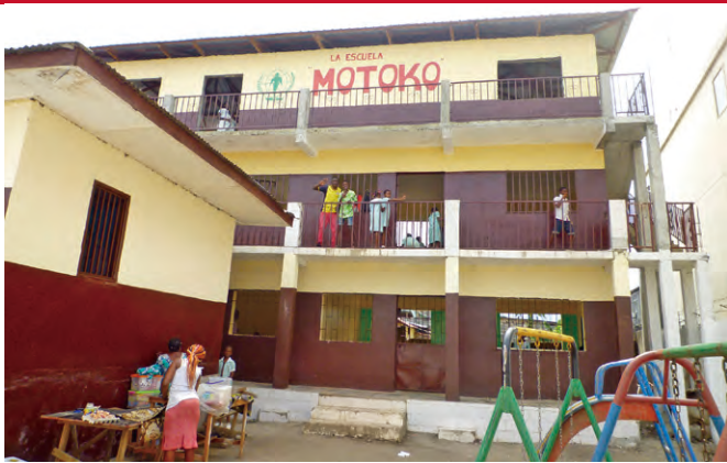
Current school building
