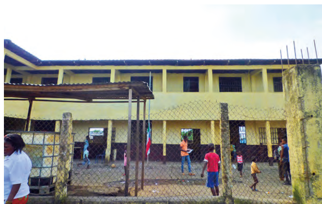
Current school building
