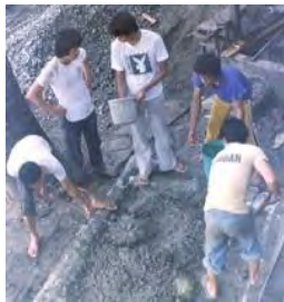
Making a cement patio
