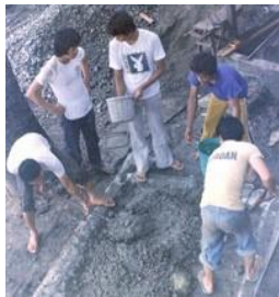
Making a cement patio
