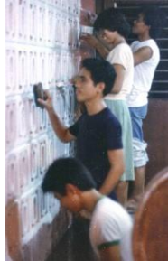
Restoring Walls inside center
