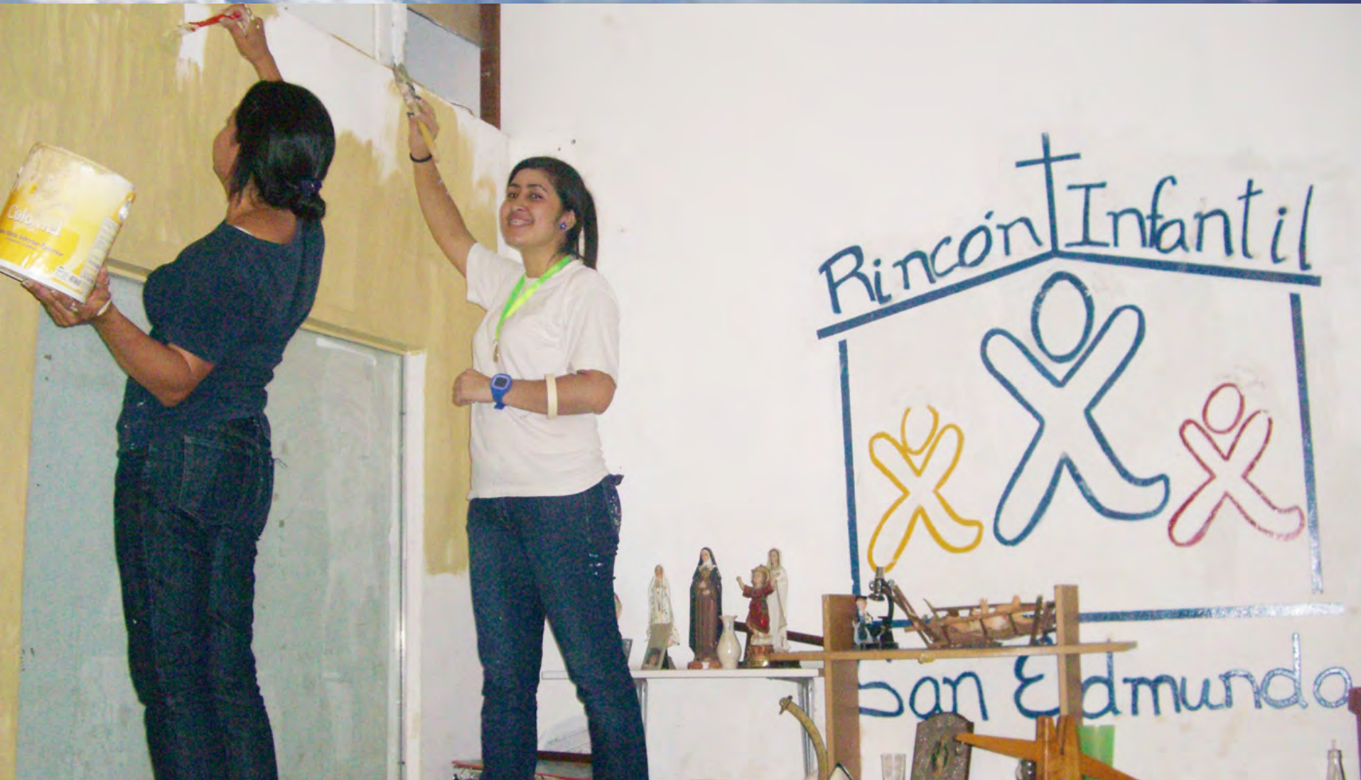
VENEZUELA: Making repairs at the St. Edmund Kids' Corner Foundation in Caracas
