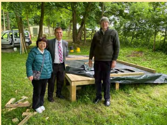
Ed Stacey is working on the new toilet block - the foundations are in
