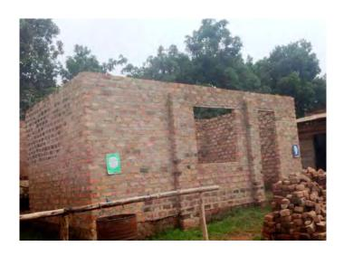
The perimeter wall, although well-constructed, requires plastering to protect it from the challenges of the weather, like heavy rain. Similarly, another structure is under construction and needs a roof in order to be completed.
