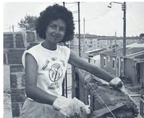
Marcia de Abreu lays bricks in the process of building a community center at site 2.
