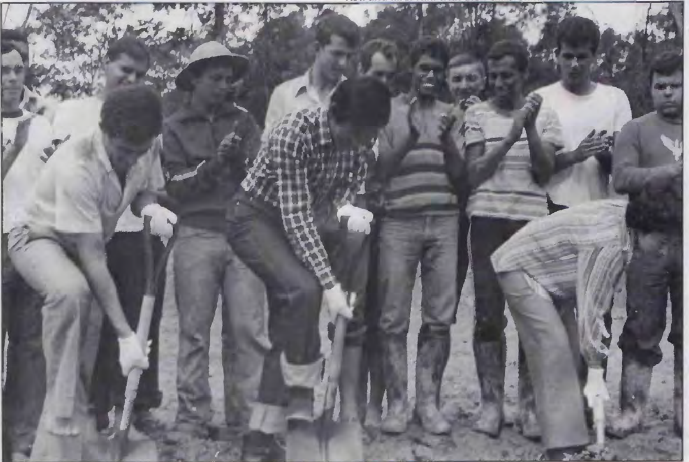
Rev. and Mrs. Kim and various state leaders, digging the foundation for a training center on recently-purchased land.
