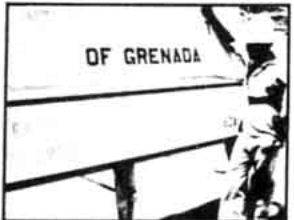
Airfield under construction in Grenada.
