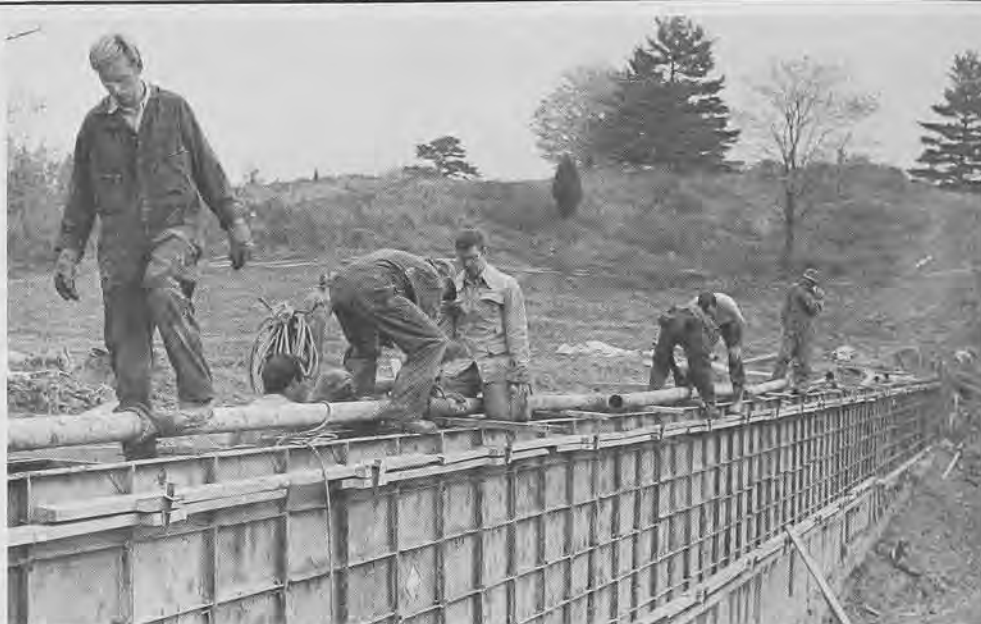
Final preparation on the frame for the new dam.
