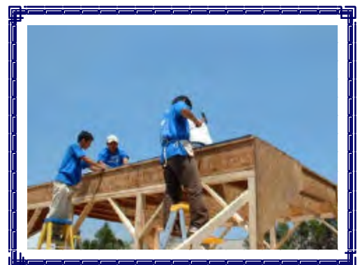
Building a Shed in Norfolk, Virginia
