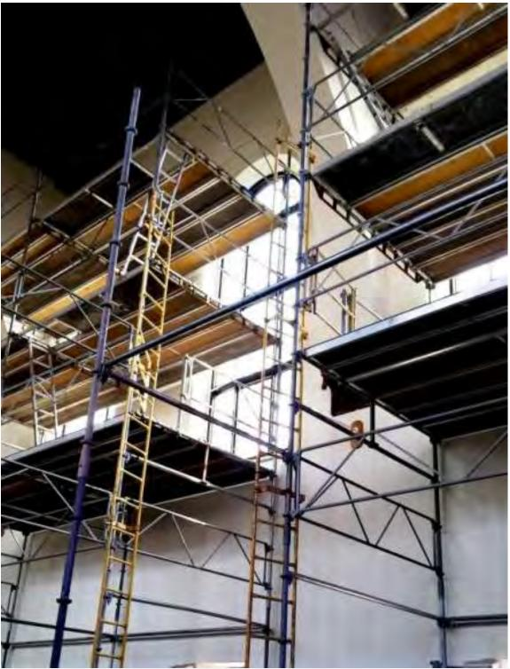
UTS Chapel with scaffolding during installation of the new, double-paned, asbestos-free windows
