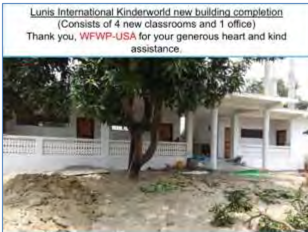
Photos of the school's construction
