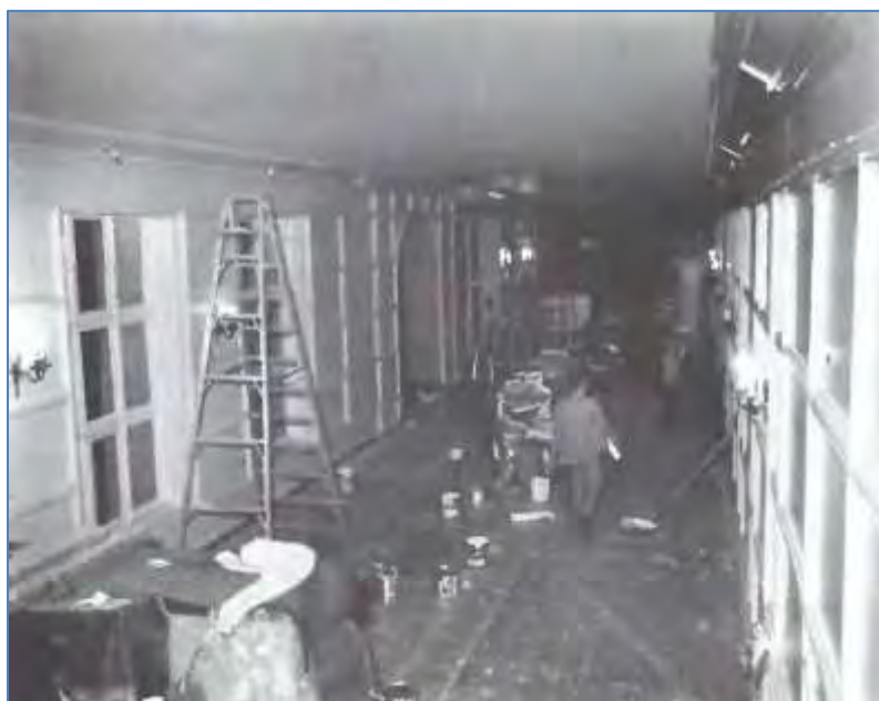
Spacious lobby required 100 man-days to paint
