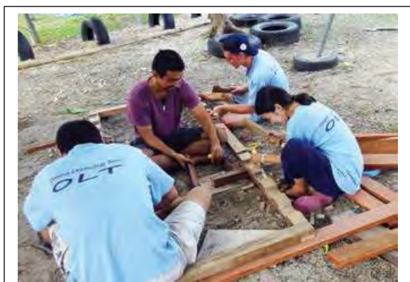
Construction for a Solomon Islands school
