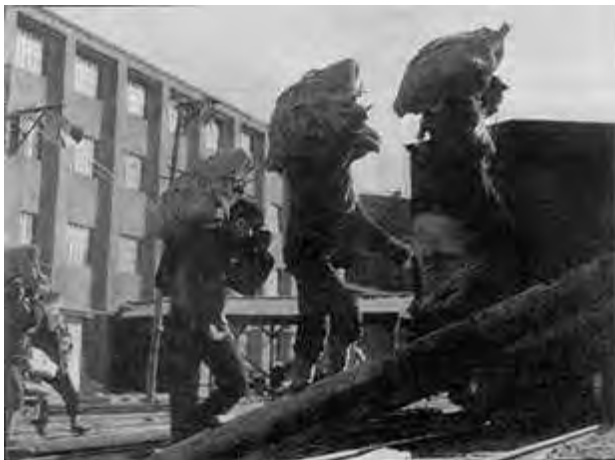
Men working at the Heungnam Labor Camp
