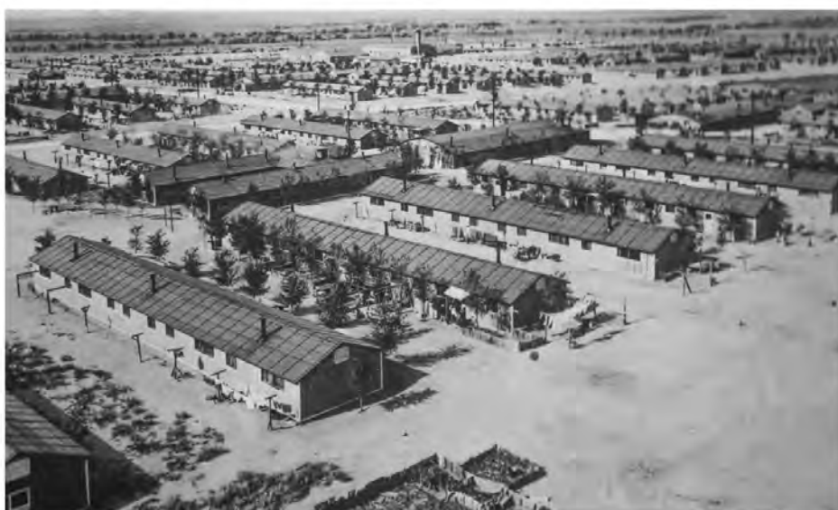
A photograph of the Amache War Relocation Center taken from the prison camp's water tower during World War II. The camp was the state's 10th largest city during that time. (Amache Museum, Special to The Colorado Sun)
