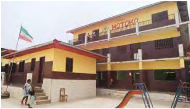
Current School Building
