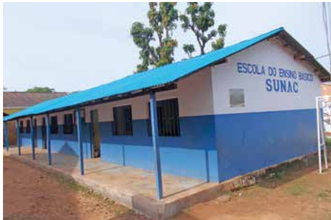
Current School Building
