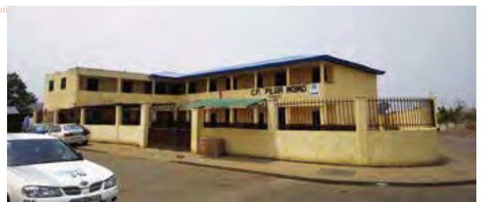
Current School Building
