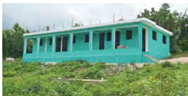
Newly Constructed School Building
