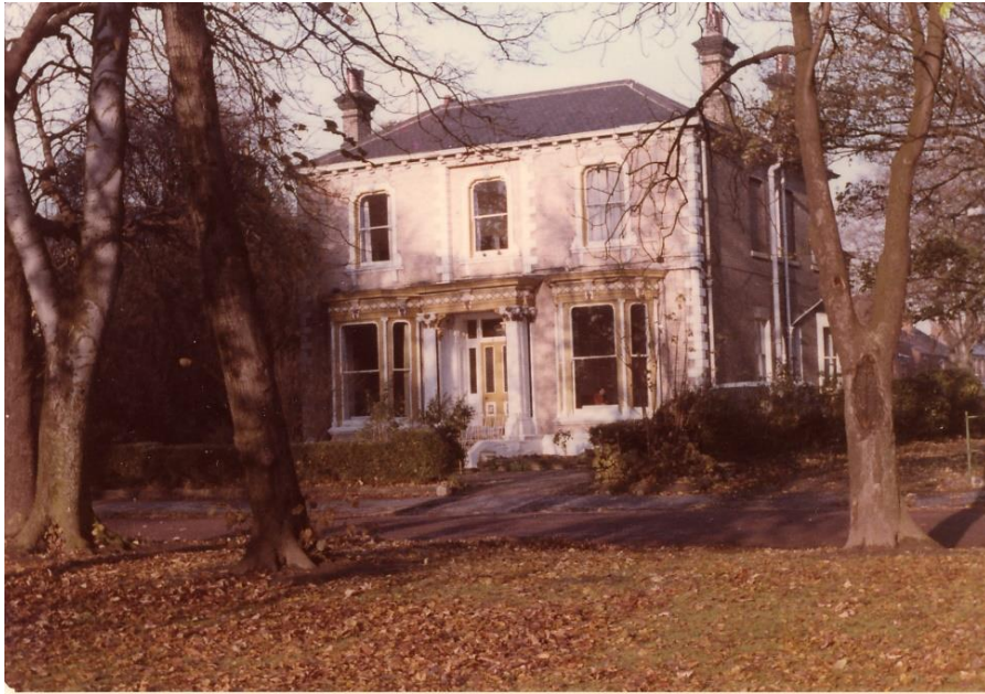
Hull Centre in Pearson Park
